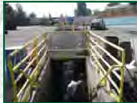
An example entrance of an underground well cellar. Matrix Oil Corporation
